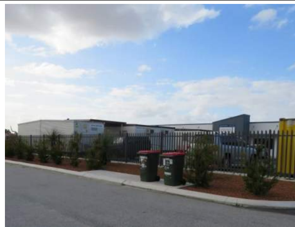
Example of landscaping in an area that experiences helicopter rotor downwash. Note concrete area for weekly waste collection. Bell Court.
