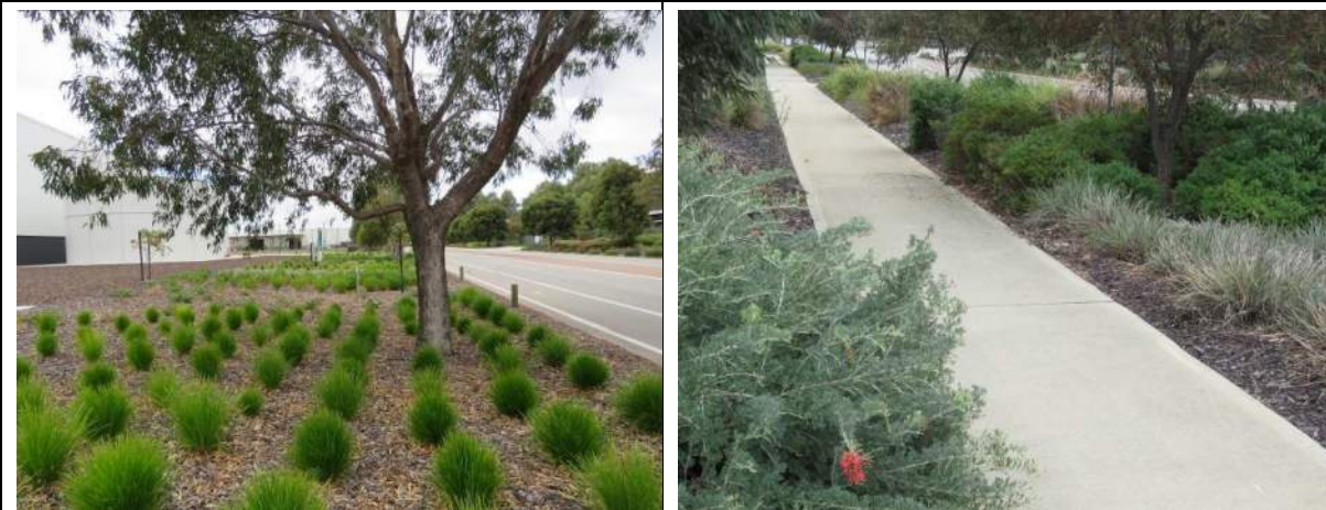
Note absence of roadside kerb/edging to allow for stormwater drainage from road, Marriott Road.
